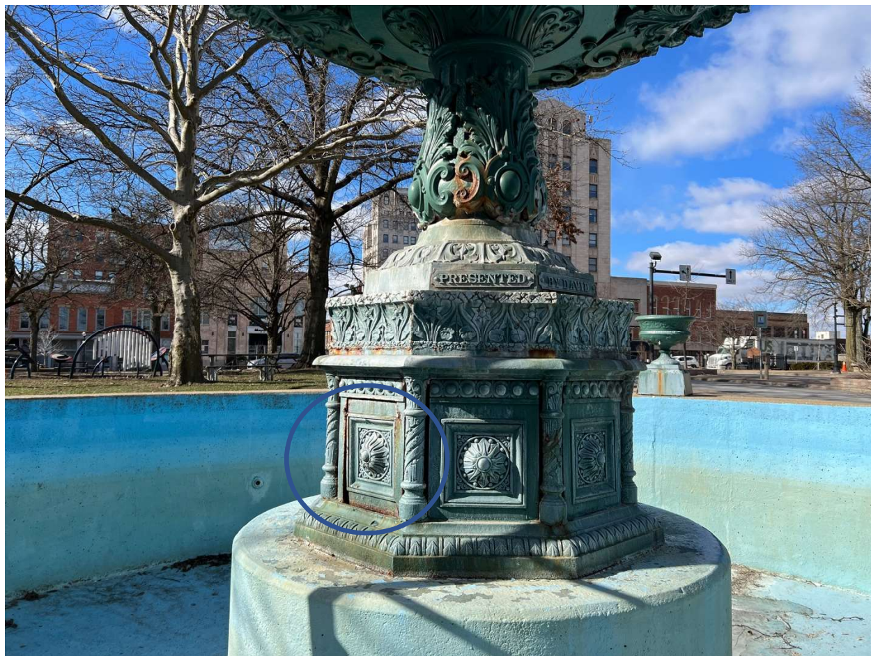
Damaged access door
