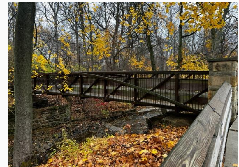
Similar construction to NLP Bridge
